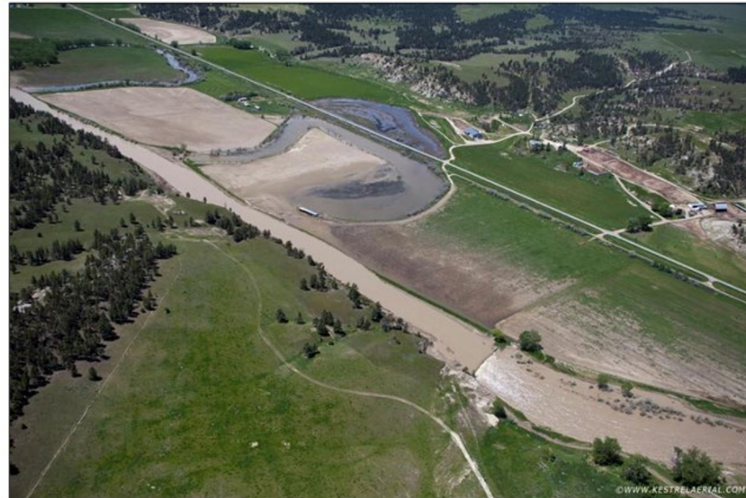
Figure 23. View upstream of Eliason Diversion Dam on June 16, 2011 showing historic channel remnants both within active corridor and beyond highway (Kestrel).
