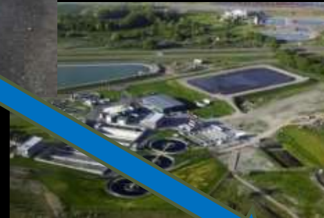
Waste Water Treatment Plant Contributing 50 kg/yr
